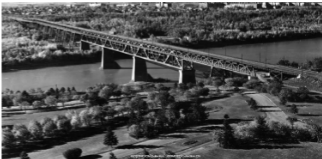
Post and Beam Bridge – built 1913
